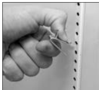
Fig. 1. Installing top tab of shelf clip.
