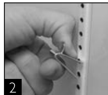
Installing bottom of the shelf clip
