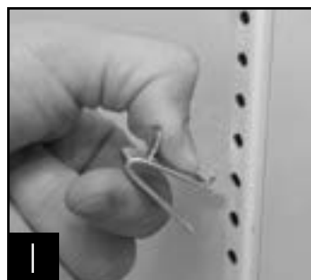
Installing top tab of shelf clip
