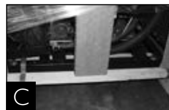
Removing skid from bottom of cabinet.
