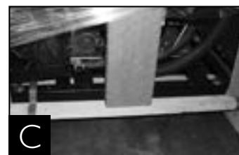
Removing skid from bottom of cabinet.
